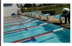
Anti-wave racing lane dividers made from 150mm diameter UV stabilized high density polyethylene discs assembled on stainless steel
