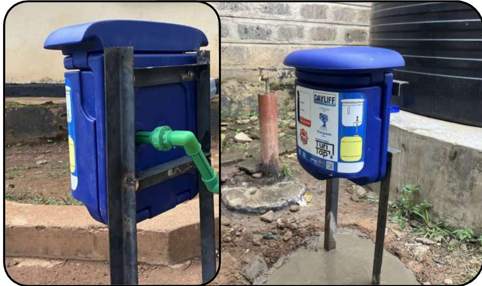
Figure 12: Example free-standing TuriTap mounted to custom frame with concrete footing
