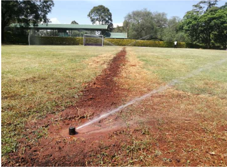
Newly installed pop-up sprinklers at one of the playing fields
